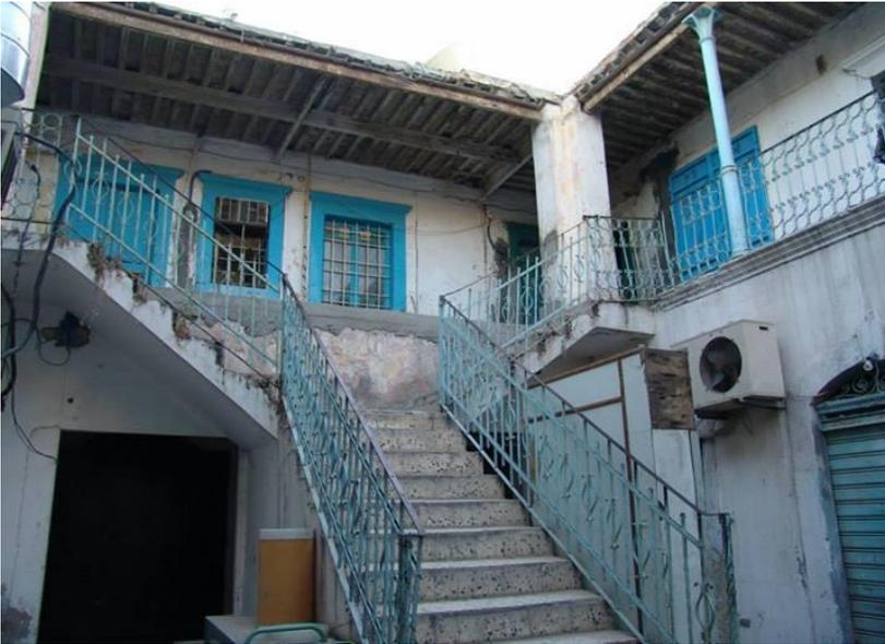
Figure 8: A house in Tripoli castle with the addition of inappropriate material and utilities
